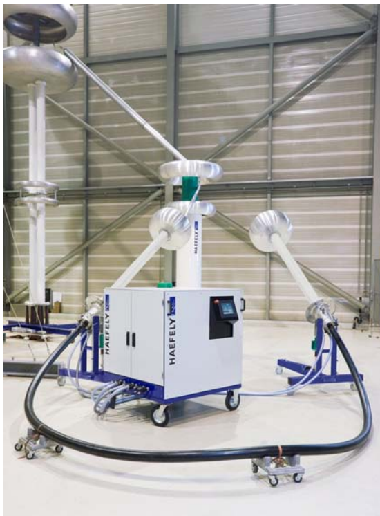
CTT & WPU with 110 kV XLPE cable
